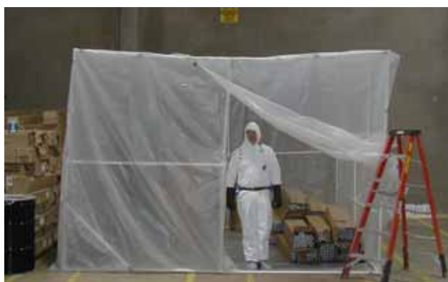
Photograph 2.2: EPSI Phoenix Facility - Containment Structure
