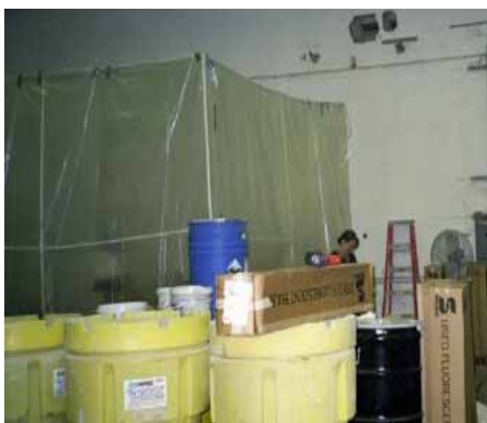
Photograph 2.3: AERC Melbourne Facility - Containment Structure
